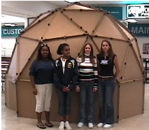
Figure 10. A completed dome with base ring.
